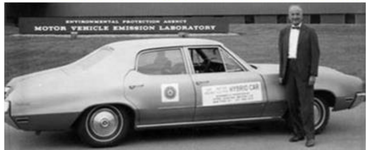
In the 1970s, Dr. Victor Wouk, an electrical engineer by training, built one of the world's first hybrid cars. Wouk effectively modified a 1972 Buick Skylark to run on both gasoline and electricity, setting the stage for hybrid cars many years down the road.
